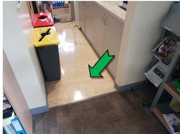
Photo 4. Interior, throughout, cream floor coverings – suspected non asbestos-containing sheet vinyl.
