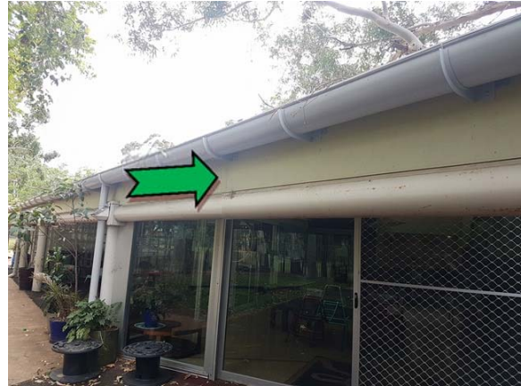
Photo 2. Exterior, throughout, fascia – non asbestos-containing fibre cement sheeting.
